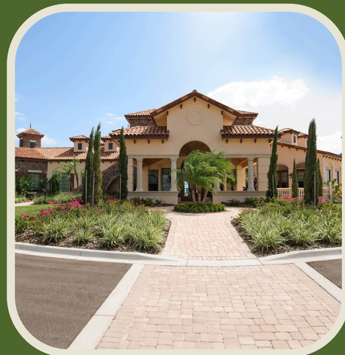
Club House Renovations
